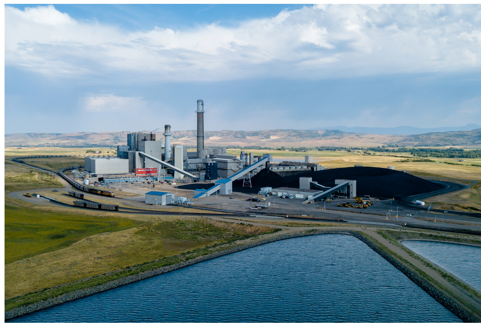
Below: Tri-State Generation and Transmission plans the early retirement of the 1.3-gigawatt coal-fired plant in Craig, Colorado as part of a statewide program to reduce carbon emissions. The transition away from coal has been a key trend over the last 15 years. (2018)
