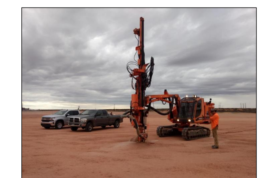
Airtrack probe drill investigation
