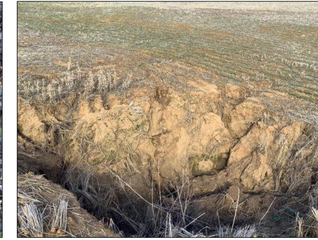
Irregular "ragged" parapet with soil raveling
