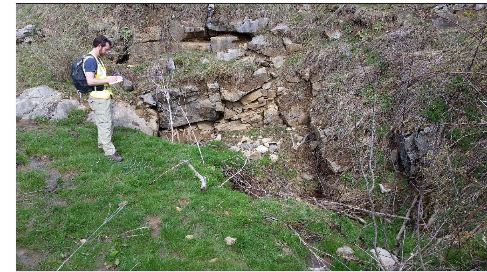
Assessing sinkhole location and characteristics
