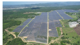
Figure 5.1: Girasol PV Plant
